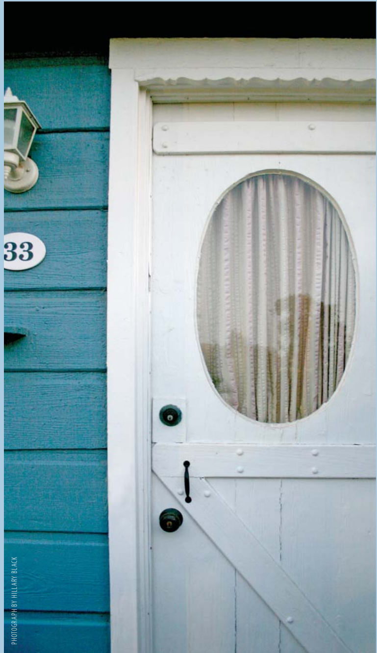
A close-up of the front door of cottage 33 shows the care and detail that went into the restoration of these historical gems.
