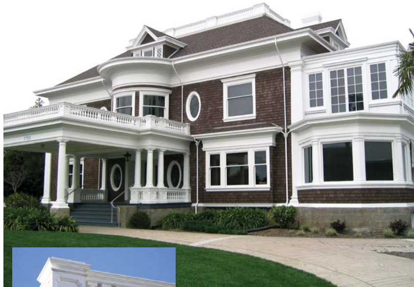
The 400 hand-turned balusters of this widow's walk, as well as the moldings, handrails and newel boxes were pre-fabricated and pre-assembled at Blue Ox, then shipped to the Noyes Mansion in Napa, California.
